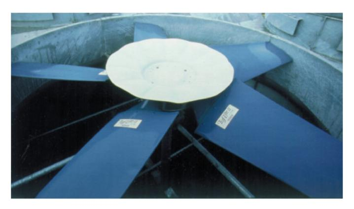
Adjustable Pitch Fan Assembly 5' through 14' Diameter
